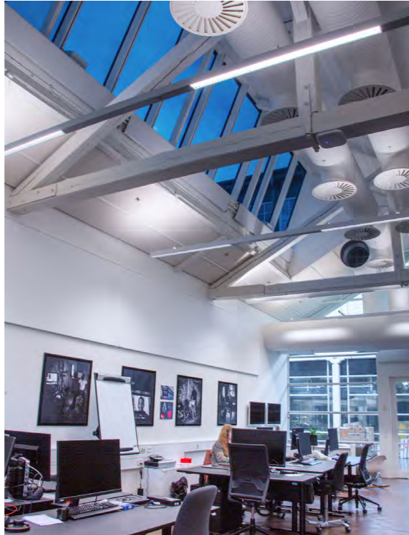
The dynamic glass' ability to change tint automatically transforms this space into an agreeable workspace. Employees can work comfortably, without being bothered by the glare or an unberable heat.
