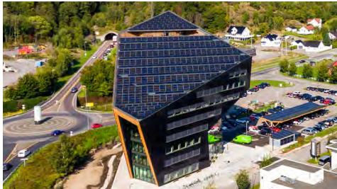
Powerhouse Telemark (Norway)
