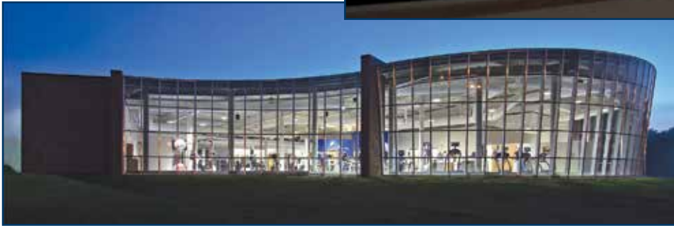
Figure 5 – Image of a large-scale installation of EC glazing at Butler County Health Care Center, David City, Nebraska. The application features a complex curved façade with glazing sloped outwards. The architects chose EC glazing because of the elegant solution to the heat and light control and the ability to maintain the views of nature on the campus for the patients in the rehabilitation center. Photo courtesy of Daubman Photography.
